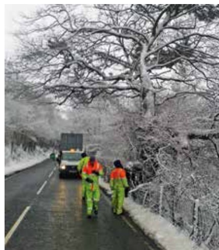
A multi-discipline approach: working with ecology and geotechnical colleagues.
